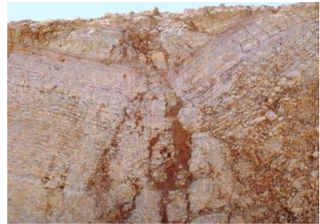
Figure 3. Exposed karst cave along rock fractures, photographed at the WAC
